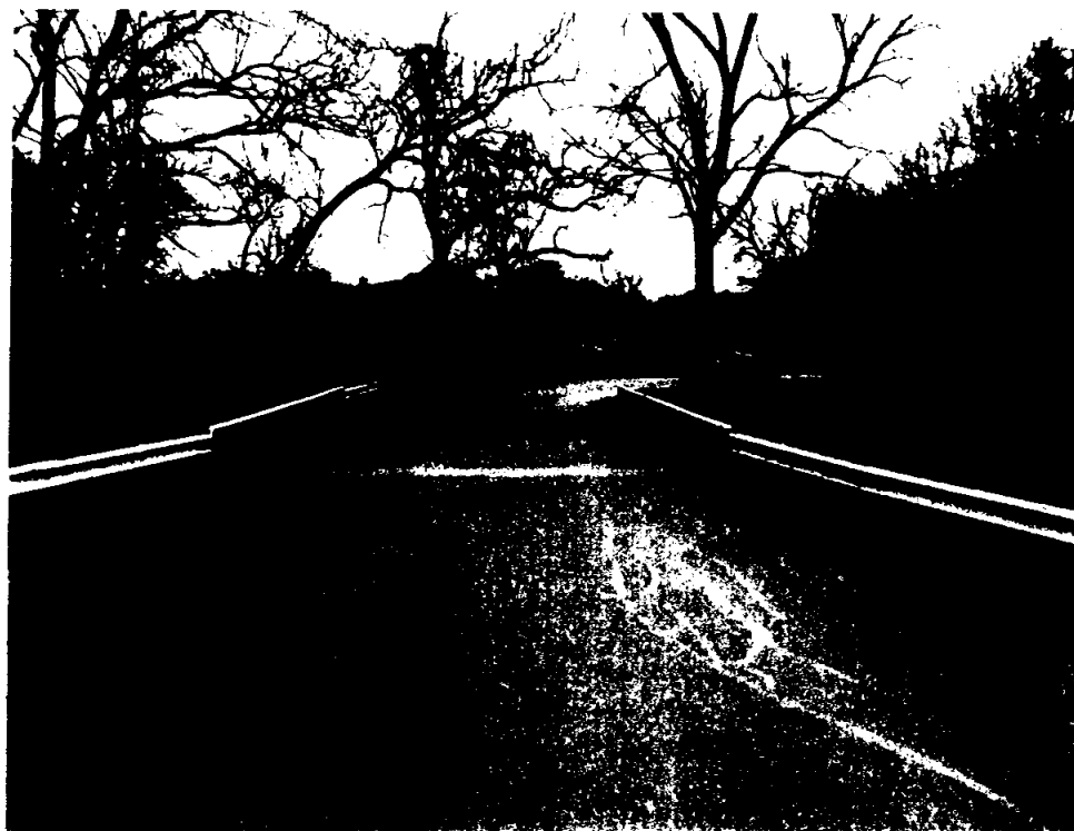
02-249-AA05-50-001 Acorn over Waggoner Branch Approach Looking South
